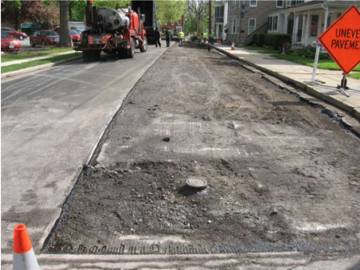
Park Place Complete Pavement Removal
