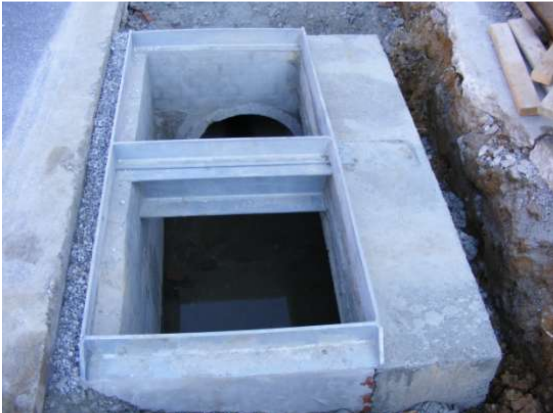
New Storm Drain Inlet - Green Street
