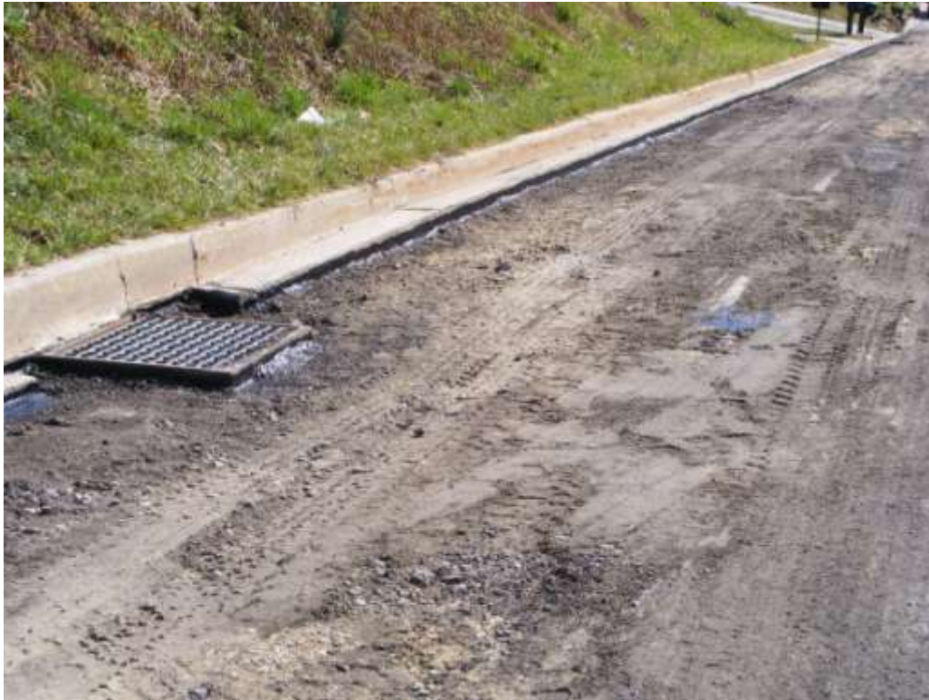
Entire Paved Section Removed
