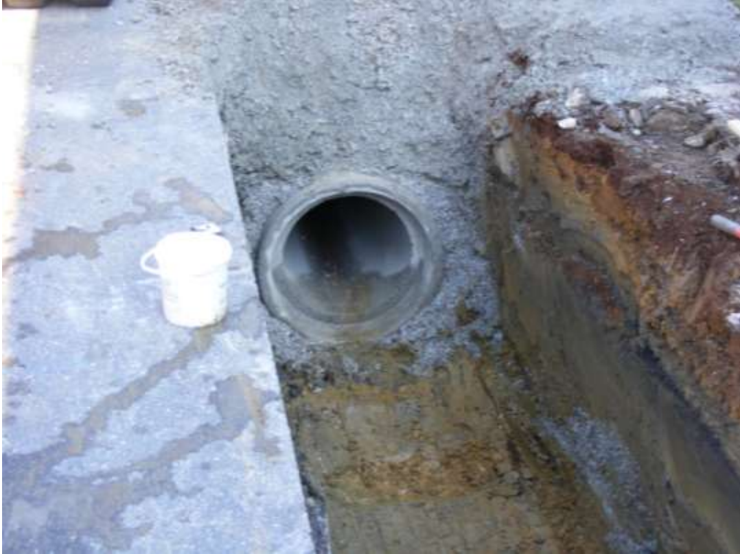
New Concrete Storm Drain Pipe - Green Street
