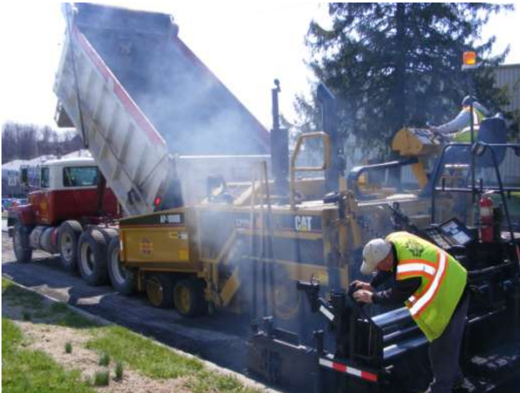
Base Pavement in Progress
