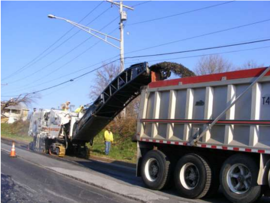
Roadway Milling in Process
