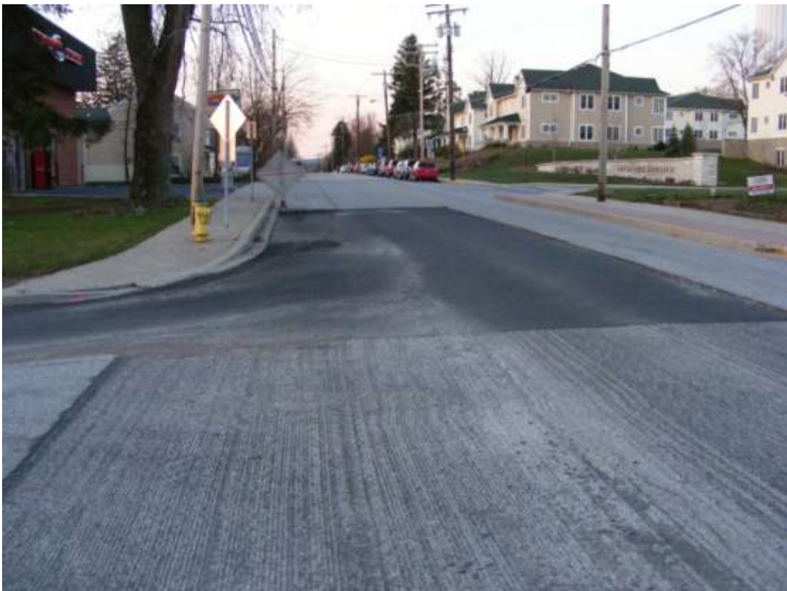
Milled Section Complete
